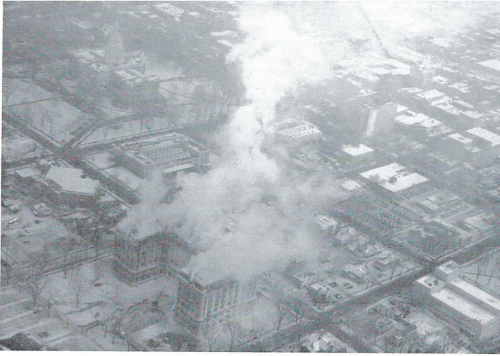
Smoke billows, firemen battle flames in this aerial picture of building.
